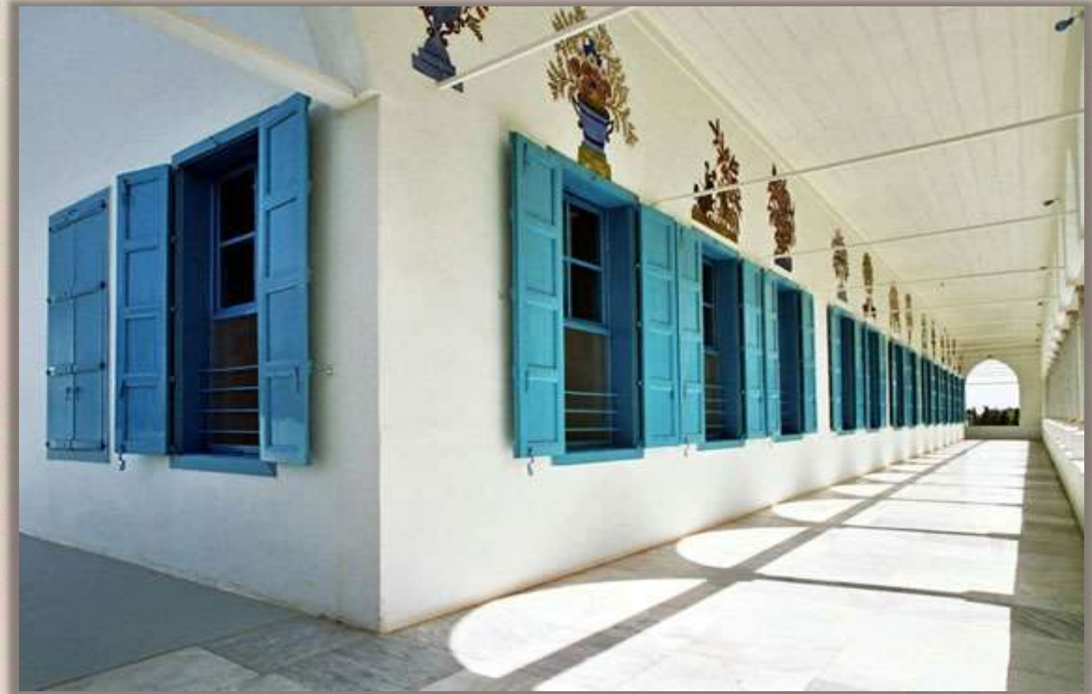
View of the southern balcony of the mansion
