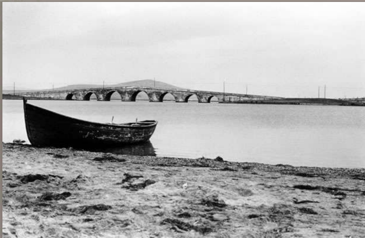
The bridge at Büyükçekmece, Turkey, which Bahá'u'lláh and His companions crossed on their way from Constantinople to Adrianople in December 1863
