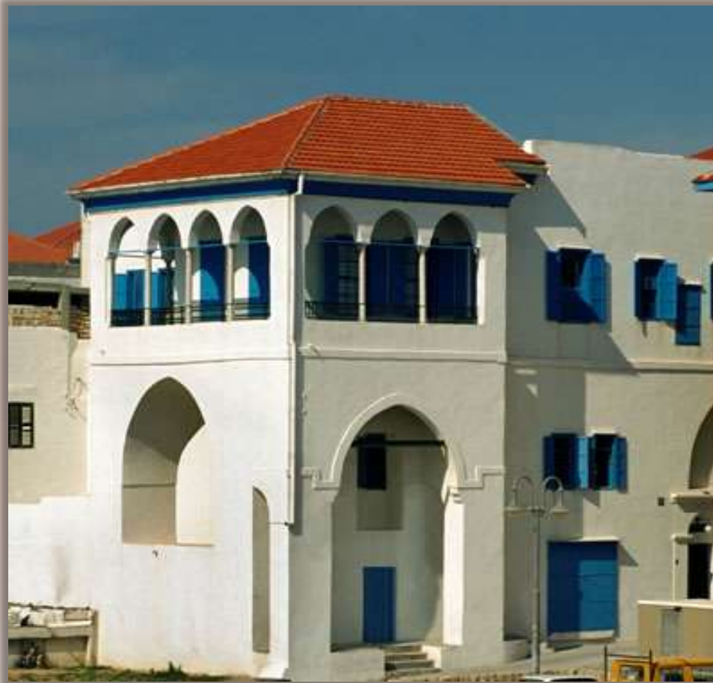
A view of the House of 'Abbúd in more recent times
